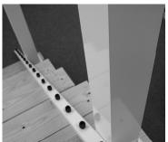
8. To mark the lines for installing the bottom rail mounts, measure down from the upper level line (from step 7) 33 1/4" for 36" rail or 39 1/4" for 42" rail on both the upper and lower posts.
